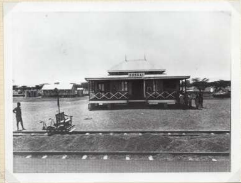
RONGAI STATION BUILDING (MILE 19 FROM NAKURU)
