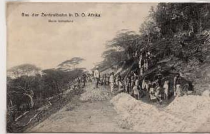
Digging out ballast (on which to lay the lines)
