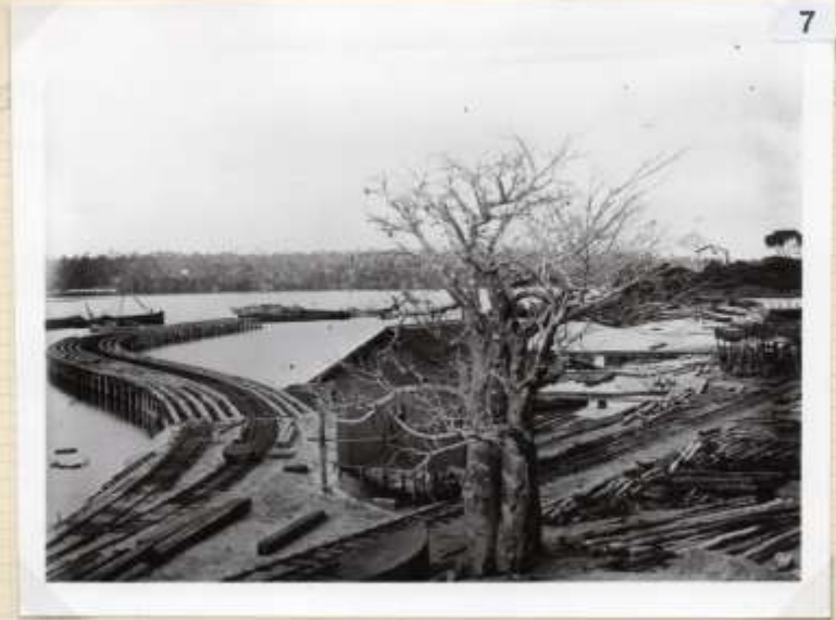
EARLY HARBOR WORKS AT KILINDINI WITH ENGINEER'S BUNGALOW.
