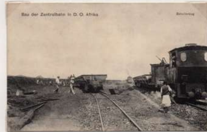
Side-tipping ballast trucks deliver the ballast on site
