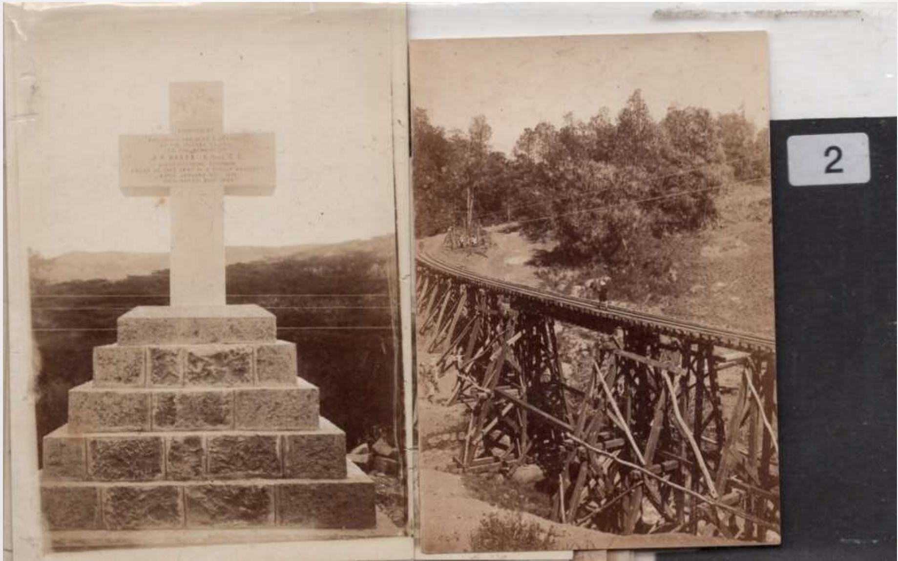
Uganda Railway – a collection of 22 sepia photographs (varying quality) including of the construction of the railway and a picture of Arthur F Church
